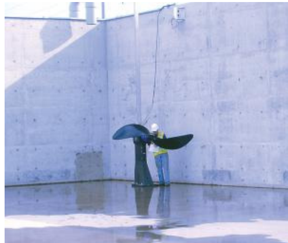
A large-blade Amaprop mixer installation from KSB is shown in and anoxic reactor at the City of Grand Island Wastewater Treatment Plant.
