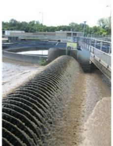
originally designed as a pre-clarification step to lower the Solids Loading Rate on the existing final clarifiers—were inefficient and interfered with channel velocity, causing mixed liquor suspended solids (MLSS) to settle in the basins. Upon evaluation by Siemens product experts, it was discovered that the existing tank widths were ideal for disc aerators.
