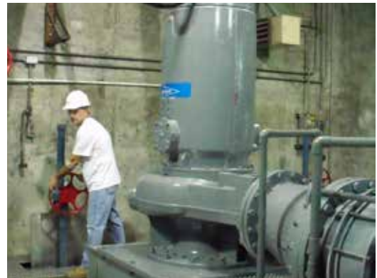
Lower level of Baltic Avenue pump station now housing one 135 HP and two 200 HP Flygt clog resistant dry pit submersibles pumps.
